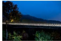
The lighting requirements included 15-lx minimum levels across the roadway surface with a uniformity of 0.88. The adjacent pedestrian and bicycle path required 11-lx levels.
